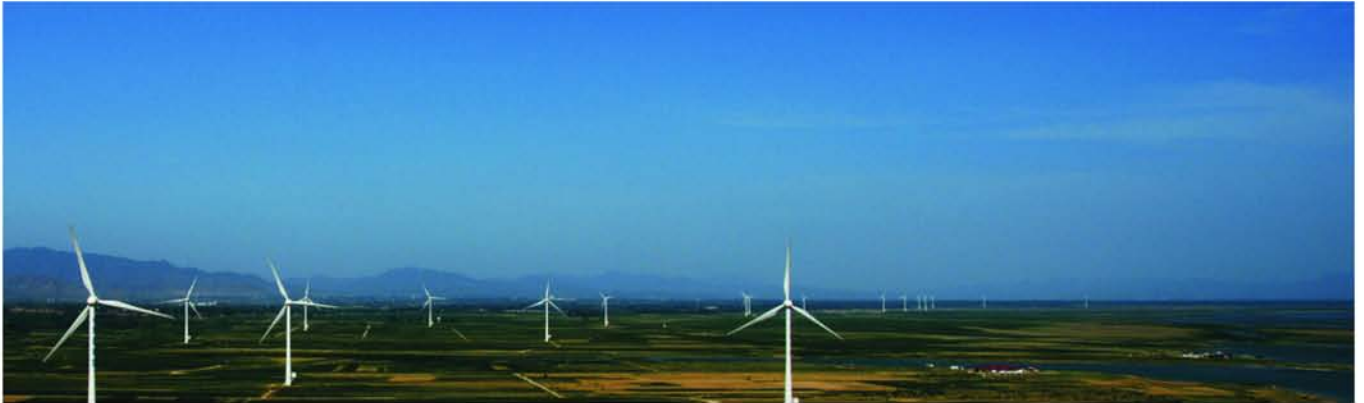
The Guanting Wind Farm
